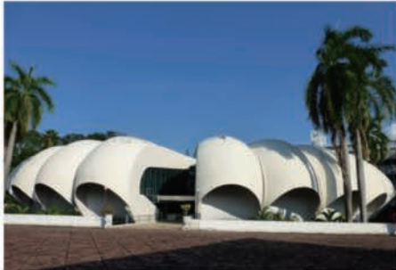
2.Lecture Center, Faculty of Science (Pumpkin building), Prince of Songkla University, Hatyai Campus, 1966; Amorn Sriwong (architect)
