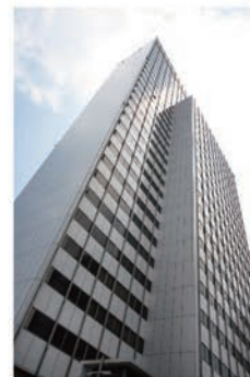
Wisma Nusantara 1966-71 KAJIMA Corporation Jakarta | Skyscraper | Office | Modernism Japanese War Reparation | Steel skeleton | Earthquake resistant experiment | Engineering | First skyscraper
