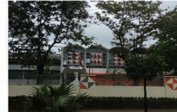
Singapore-Myanmar Vocational Training Institute, Yangon 1956 Raglan Squire School's 4 wings 8 storeyed hostels - the highest buildings of the time Exudes the spirit of a newly independent nation
