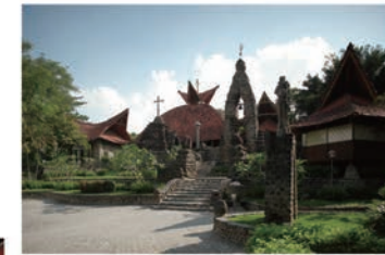
Puhsarang Church 1936 Henri MACLAINE PONT Kediri | Colonial | Catholic pilgrimage church | Terrace structure using roof tiles | Craftmanship Incorrect restoration | Masonry | Brickwork | Addition
