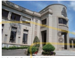
Council for the Development of Cambodia 1937 Unknown architect, French? Well preserved One of the 3 main art-deco buildings of Cambodia. It is beautifully decorated with terrazzo, metal windows and doors with high ceiling.
