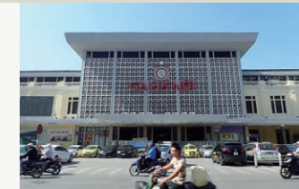
90 Central Wing of Hanoi Central Station
