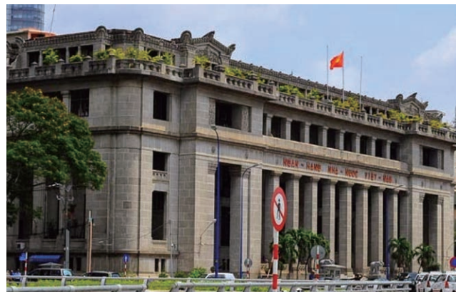
Fig2. Indochina Bank, eclecticism with Cham and Khmer expressions Elevations, columns, nest fence, steel doors, corridors, balcony, details of the roof, etc: patterns of lotus, vines, leaves, bird-head
