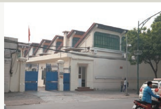
45 Postal Facility Workshop
