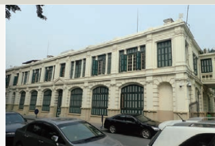
69 Office of Hanoi Municipal 12 Lê Lai, Lý Thái To, Hoàn Kiếm 1898, Renovated 1903, Bank, Charles Lichtenfelder
