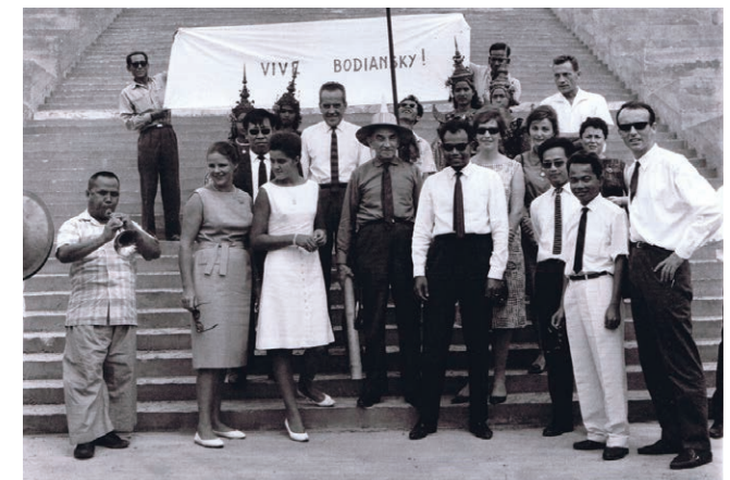
Fig.4 Bodiansky and Molyvann at the building site
