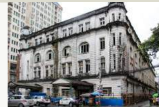
72 Former Myanmar Oil and Gas Enterprise Headquarters (Burmah Oil Company)
