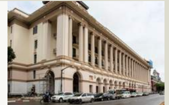
84 Yangon Division Office Complex (New Law Courts, Police Commissioner's Office)
