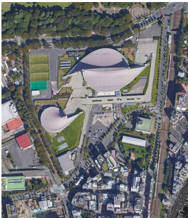
Fig.4: Aerial photo of the site and the Yoyogi Sports Complex
