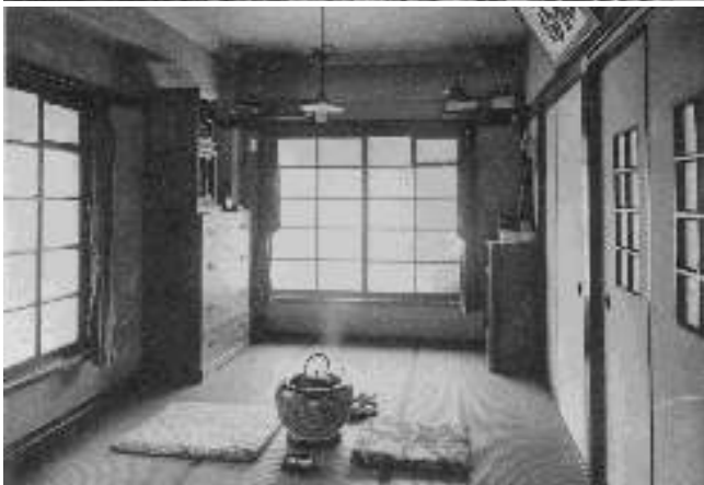
Fig.4: Outside and Inside of Dojunkai Apartment Houses (1924-1941)
