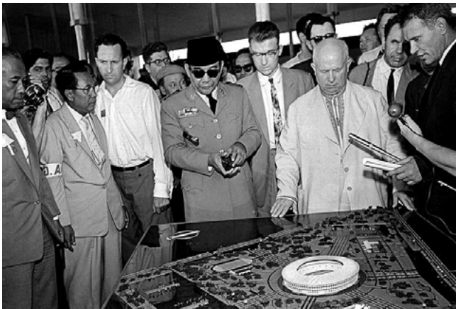
Fig.5: Nikita Khrushchev and Soekarno visited the construction site of Gelora Bung Karno sports complex (1960)
