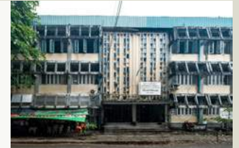
90 Yangon Electrical Power Building
