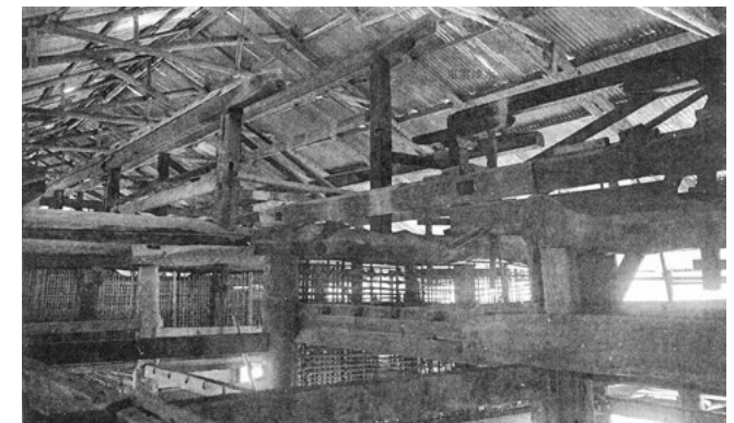
Fig.6: Tabasami-gasshoumumi (reinforced principal rafter frame)
