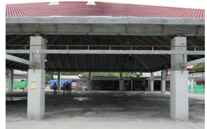
Fig.10: Cafetorium after increasing building height by extending the length of concrete column
