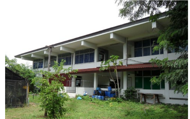
Fig.8: Exterior of former dormitory building which was changed into classroom building
