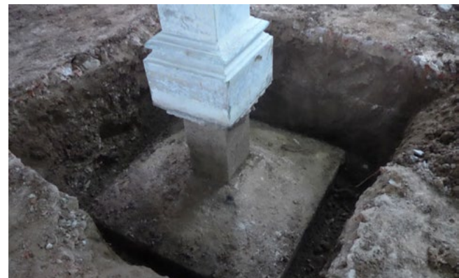
Fig.7: Isolated footing of foundation system
